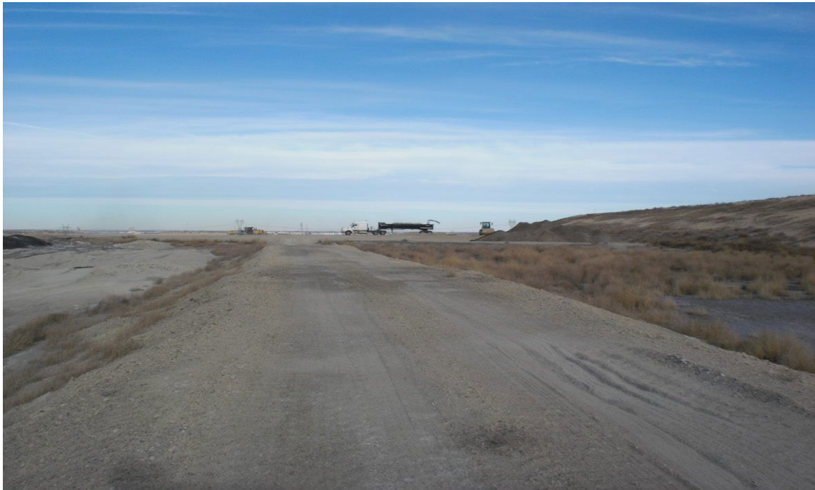
Photo 2: Phase 3A looking east. On top of waste pit.
