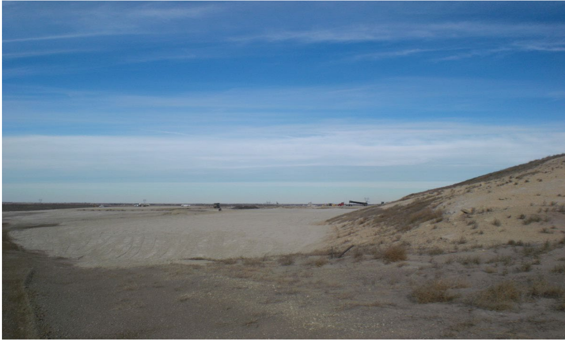
Photo 1: Entrance Road to Phase 3A
