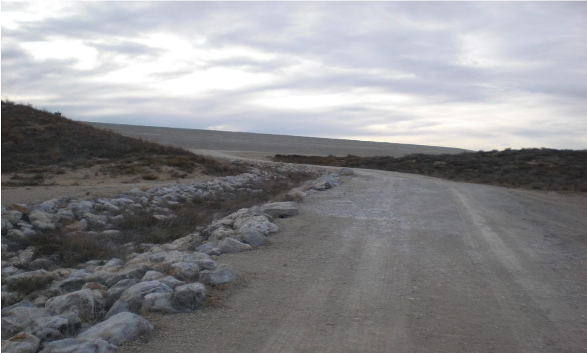
Photo 3: Contact water ditch for Landfill looking west
