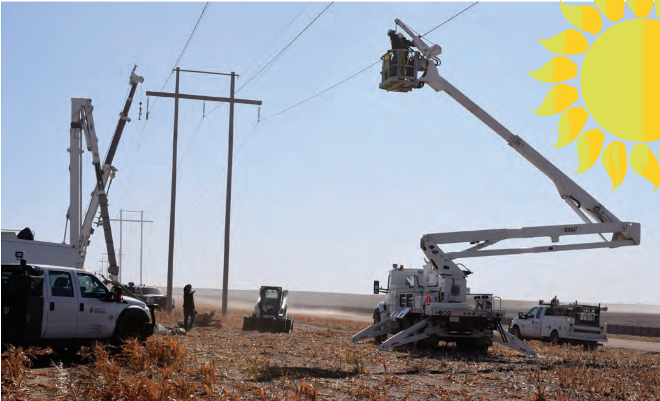
Above: Crews from Sunflower and Pioneer Electric Cooperative work together as they upgrade the line with new insulators south of the Johnson Corner Substation on Nov. 14, 2019, in Stanton County. The line voltage will be upgraded from 69 kV to 115 kV.
